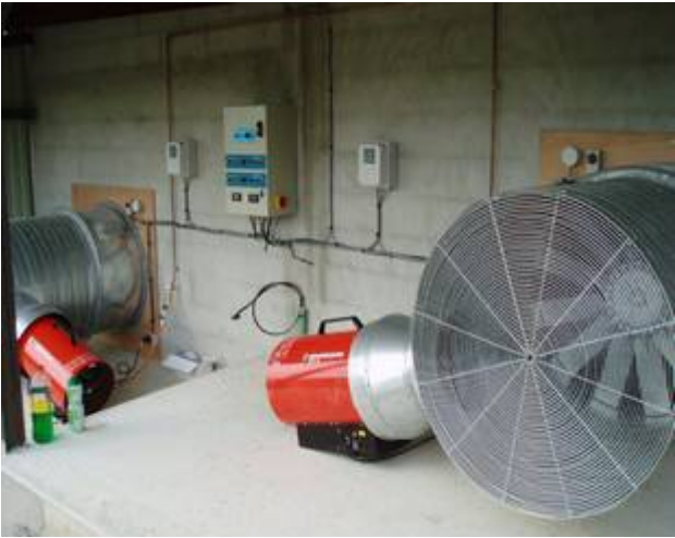
Two separate corridors, with control switchboard boxes.
