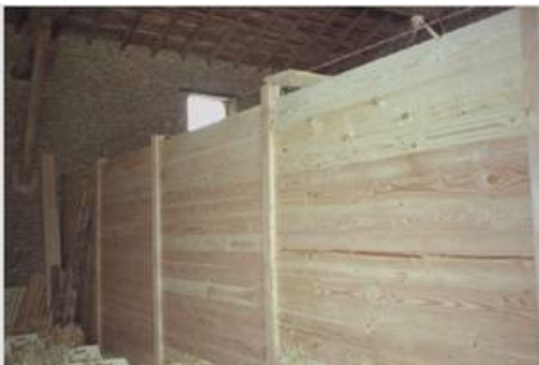
Partition wooden walls for making drying corridors:
